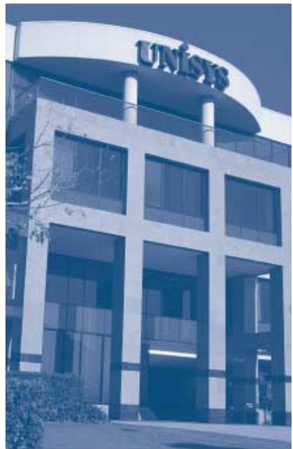
Unisys Building: current premises of the Crime function of the CMC at Milton. The function is to move to Terrica Place in 2003.
