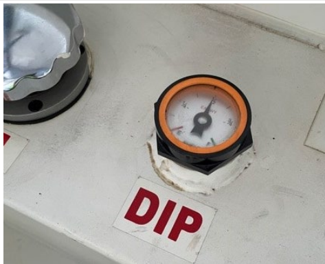
An automated fuel dip gauge to show stock level (similar to the fuel gauge in a motor vehicle).
