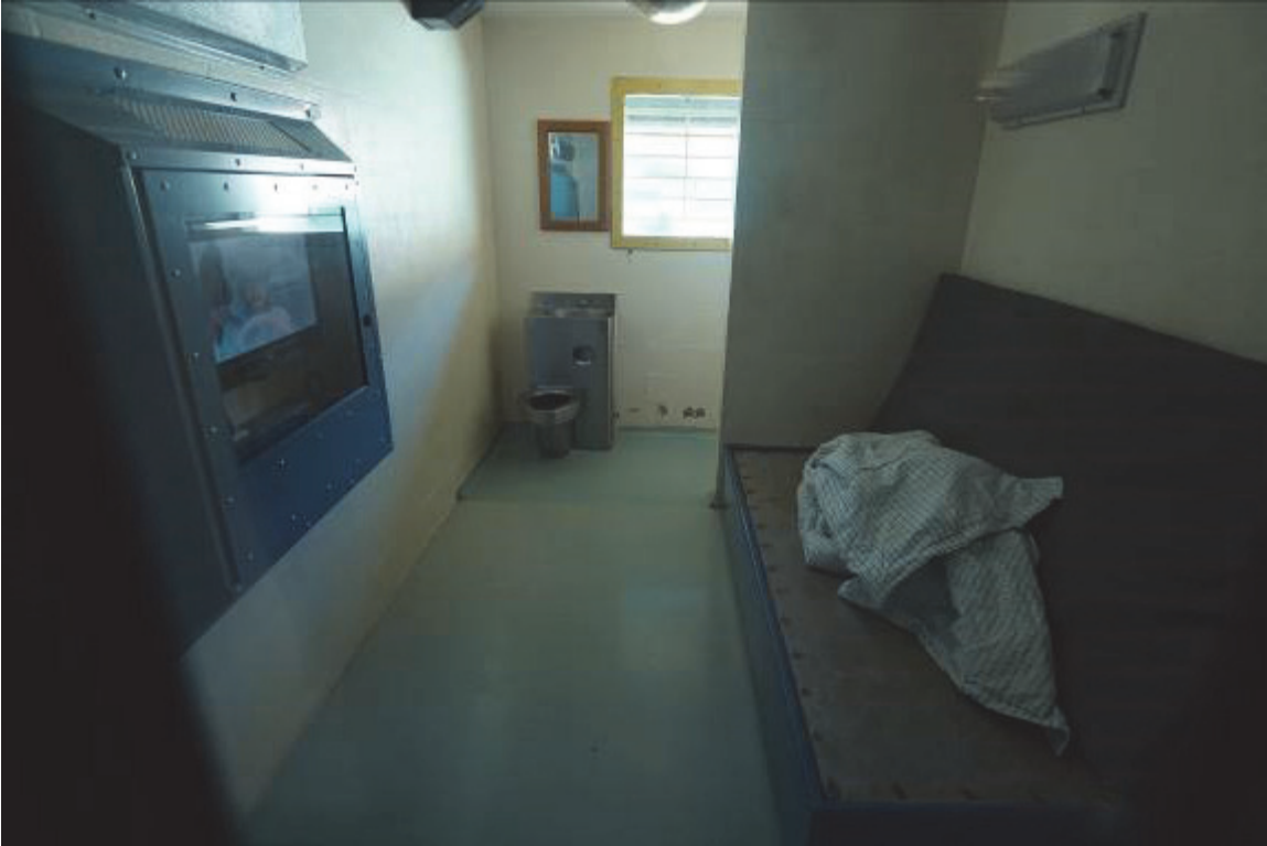
A solitary confinement cell located in the safety unit of Brisbane Women's Correctional Centre in Queensland. The cells are designed with CCTV cameras; no ligatures, hooks, or sharp edges; furnishings are bolted to the ground or flush to the wall to minimize risk of self-harm.
